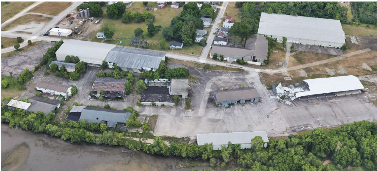
Figure 1. Aerial photography depicting significant structural damage to buildings requested for removal. (Photo taken from Google Earth Pro).
