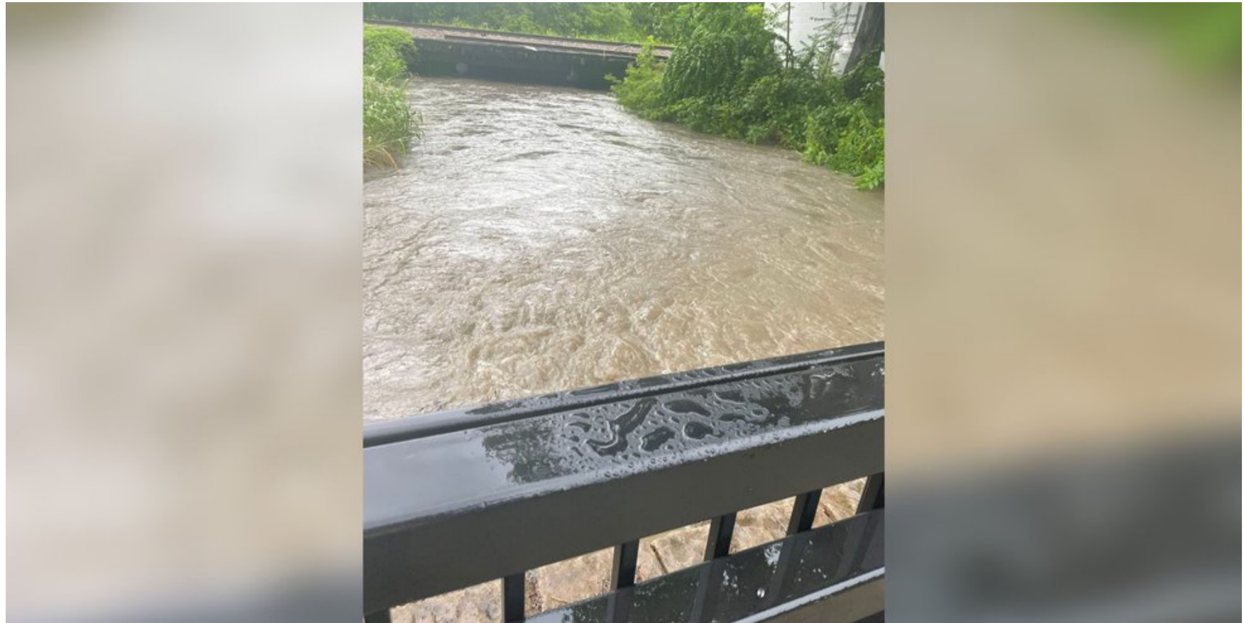
Flooding on Bollingbrook Street in Petersburg (City of Petersburg)
