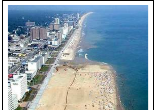
This photo, taken while the Virginia Beach Erosion Control and Hurricane Protection Project was underway, shows the significant difference between the unimproved area and the area of the widened beach berm already completed.
