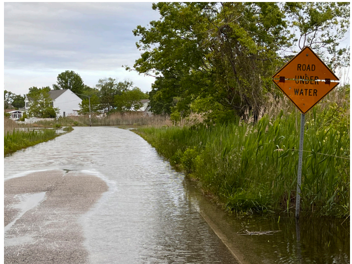
Lowest Stretch of Fifth Street During Tidal Flooding Event
