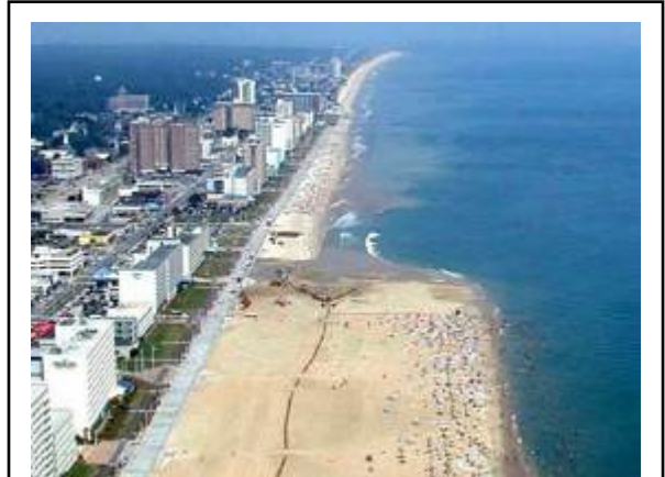
This photo, taken while the Virginia Beach Erosion Control and Hurricane Protection Project was underway, shows the significant difference between the unimproved area and the area of the widened beach berm already completed.
