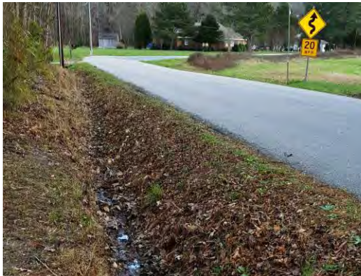
Typical rural roadway with ditch in Virginia Beach
