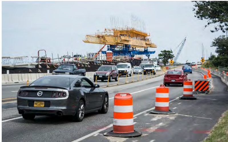
Construction of new Lesner Bridge Replacement over Lynnhaven Inlet
