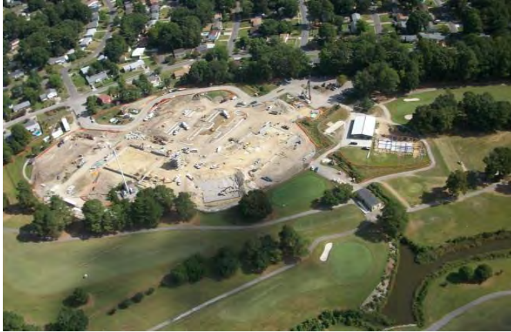
Bow Creek Recreation Center and Golf Course – before renovation
