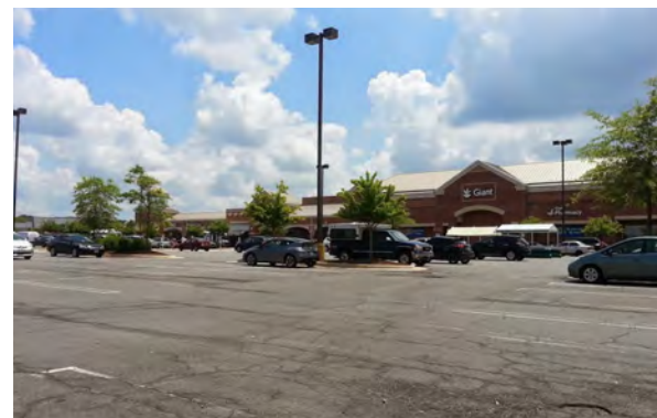
Some older retail centers lack the character that contributes to the desired Leesburg brand.
