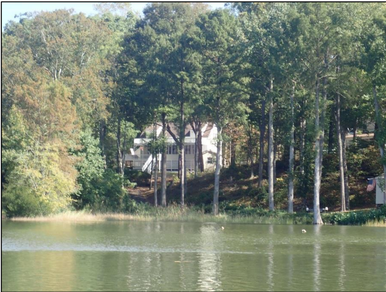
Image 3. A home that's close to the edge of Grays Creek.
