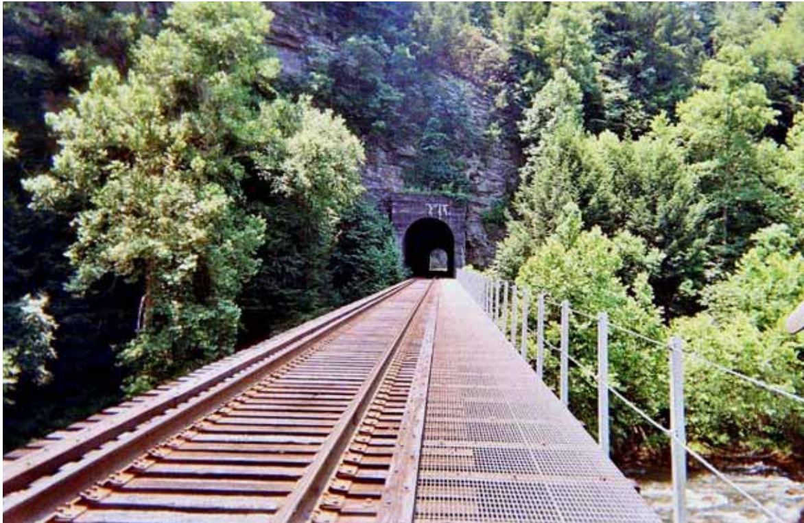
3 Skegg Tunnel – railroad bridge with pedestrian walkway for miners to get to work
