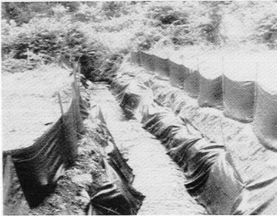
A Diversion Channel may be utilized to allow "work in the dry".
