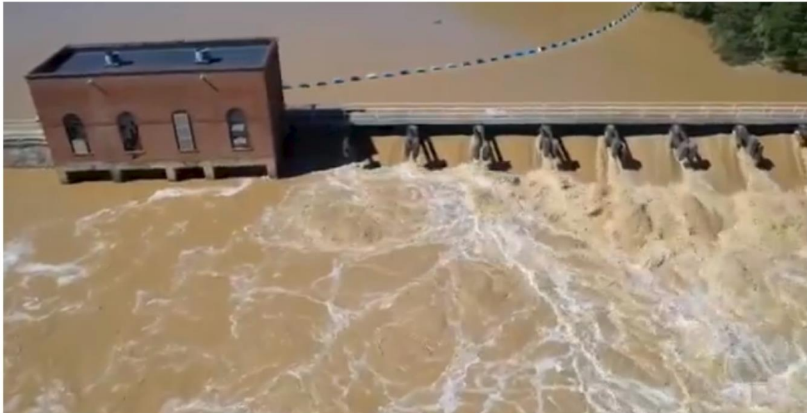
October 2018: Banister Dam is nearly overtopped following Tropical Storm Michael
