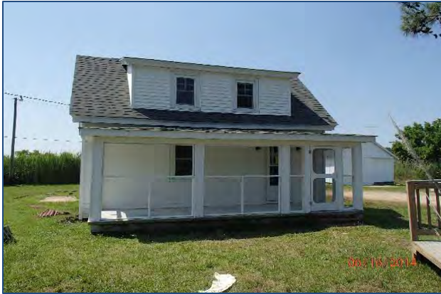
Figure 75: House in Hayes, Gloucester County - BEFORE elevation.
