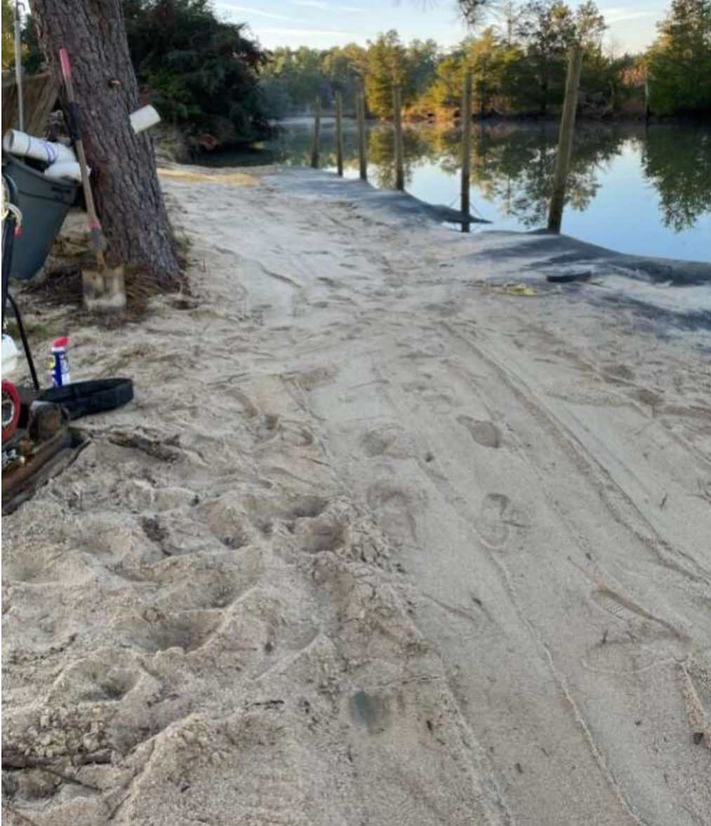
Figure 9: Recently permitted and constructed project utilizing geotubes filled with dredged material in Gloucester. The picture shows the tube as it is being covered with sediment. Grass has since been planted atop the tube and the site will function as a docking area at a public boat landing.
