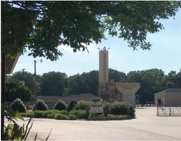
Rappahannock Concrete Corp along Route 17 - Source: Gloucester Planning and Zoning
