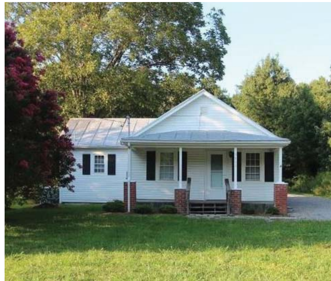
Example of older home in Gloucester County - Source: Gloucester Planning and Zoning
