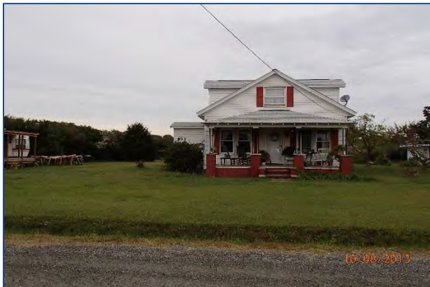
Figure 79: House in Hayes, Gloucester County - BEFORE elevation.
