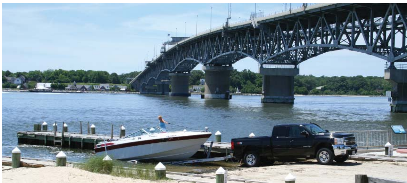
Gloucester Point boat ramp - Source: Gloucester Parks, Recreation & Tourism
