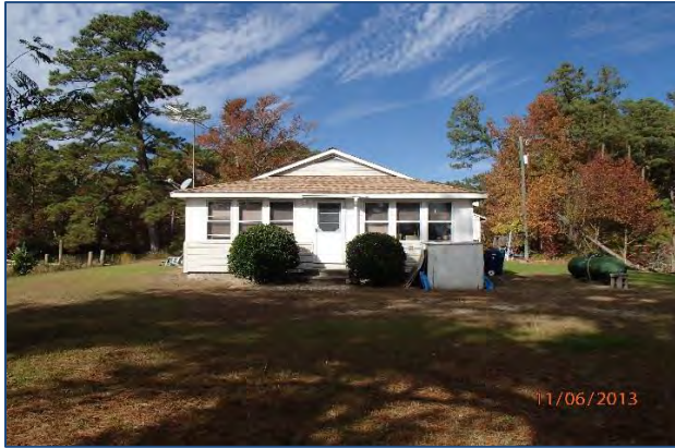
Figure 77: House in Hayes, Gloucester County - BEFORE elevation.
