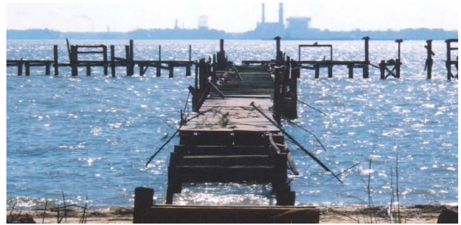
Damage to Gloucester Point pier during Isabel - Source: Gloucester Parks, Recreation & Tourism
