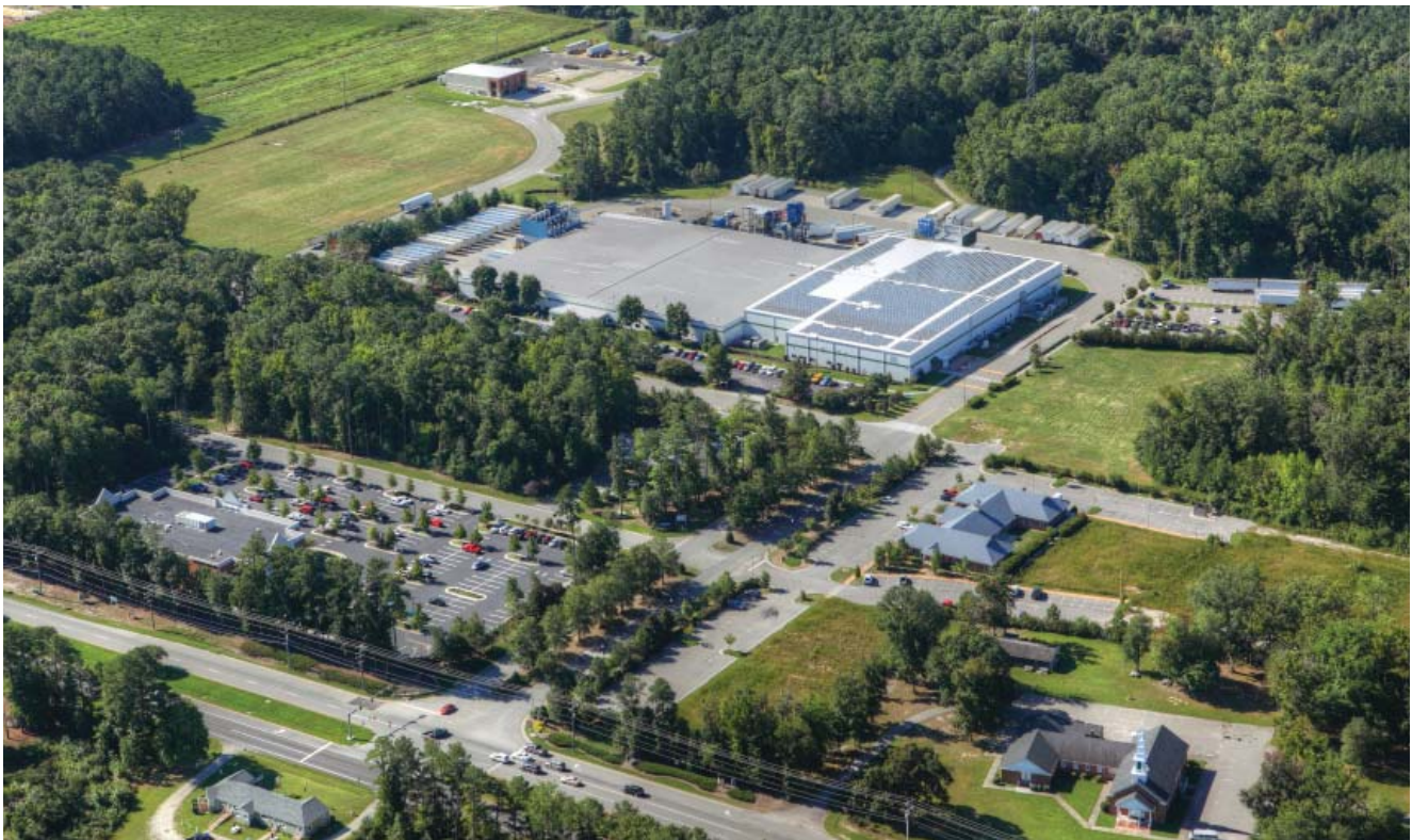
The Gloucester Business Park, a 70-acre development located south of the Court House - Source: Gloucester Economic Development
