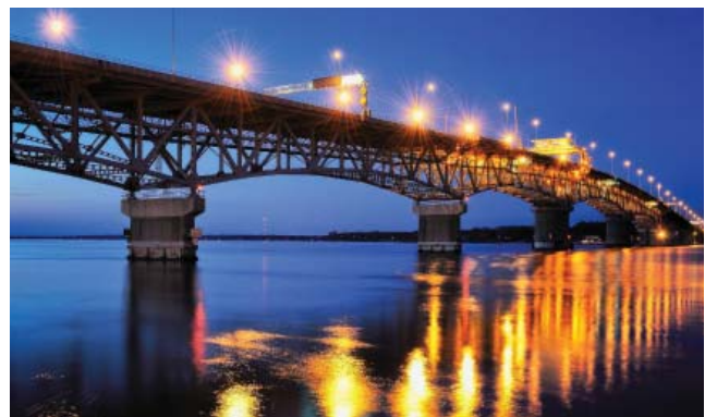
George P. Coleman Bridge - Source: William Thomas, Virginia Beach
