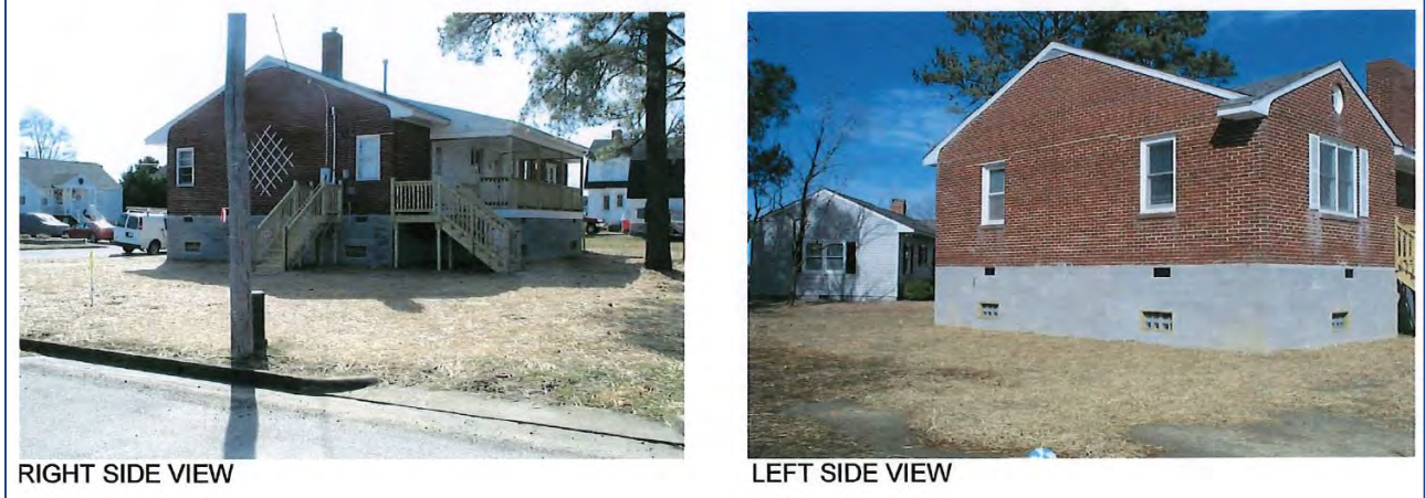
Figure 84: Photos of a home in the Town of West Point after being elevated.
