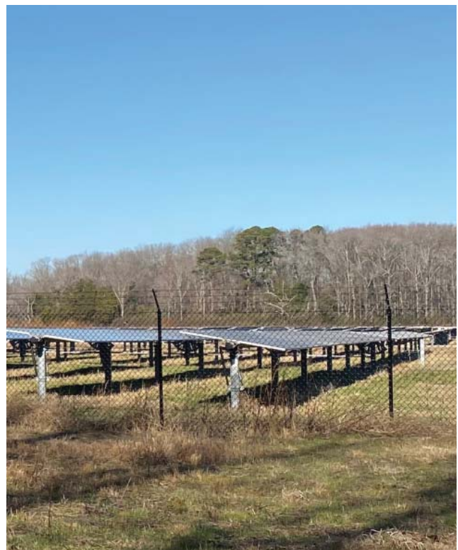
Gloucester Solar Electric Power Plant - Located off Rte. 14, the first Board approved utility-scale solar energy facility within the County.
