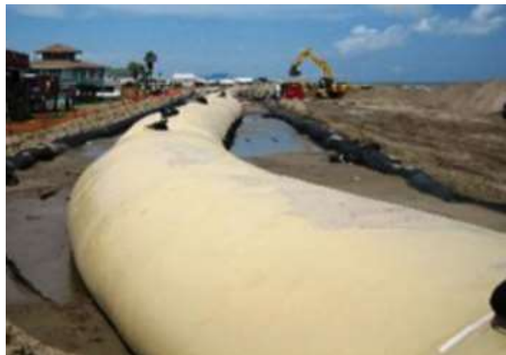
Figure 4: Example photo of a Geotube® used for sediment containment. Note that the proposed design will call for the tube to be covered with sediment and plants unlike what is shown here. (Source: TenCate website)
