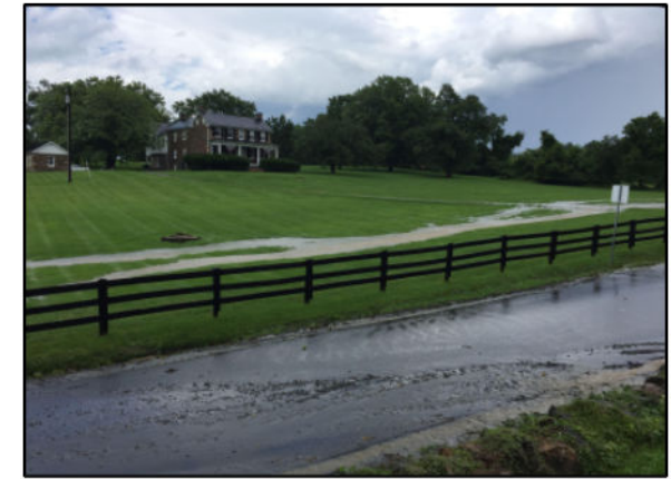
PHOTO 2 FLOODING ON WATER ST.
