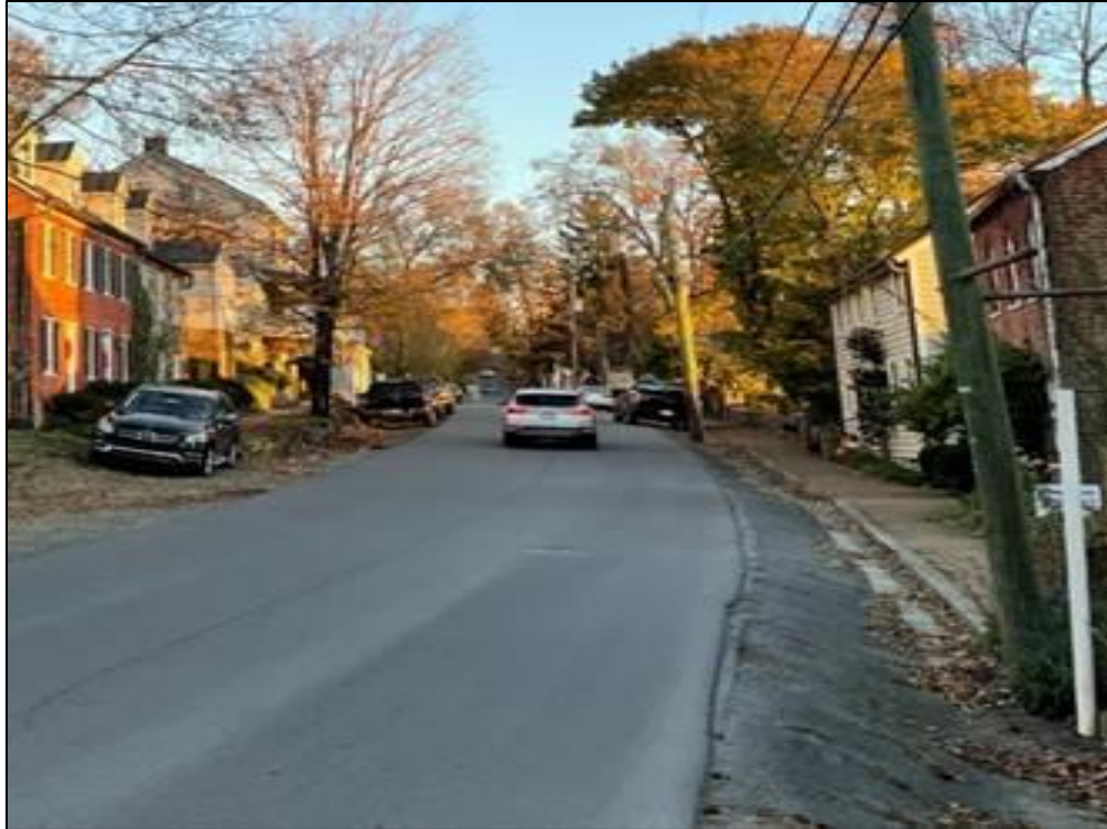
Photo 7. Lower Main Street Drainage Pattern and lack of drainage infrastructure.
