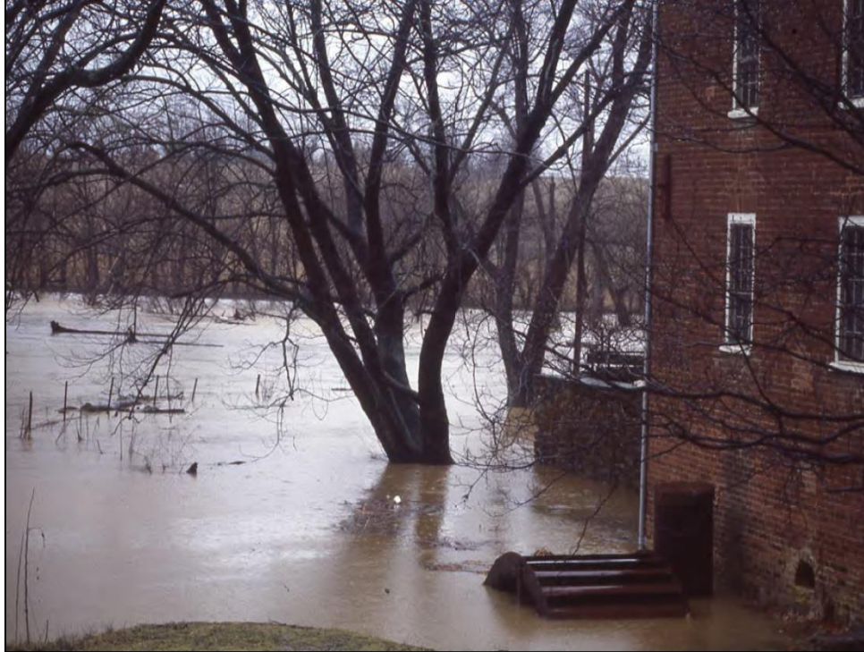
Photo 1. South Fork of Catocin Creek flood impacts on the Waterford Mill.
