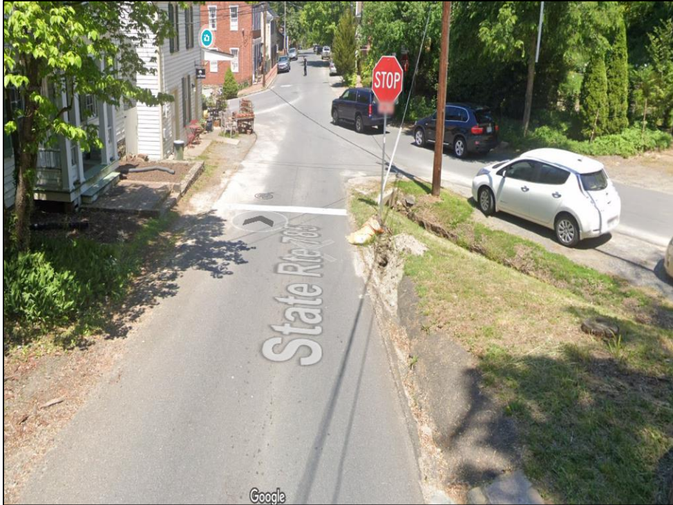
Photo 5. Sandbag Implementation and inadequate drainage infrastructure at the intersection of 2 nd Street, Water Street, and Main Street.
