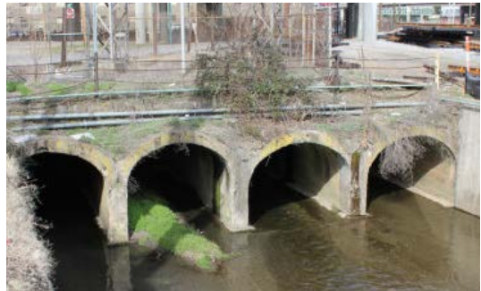
Figure 1-2: Tunnel Outfall
