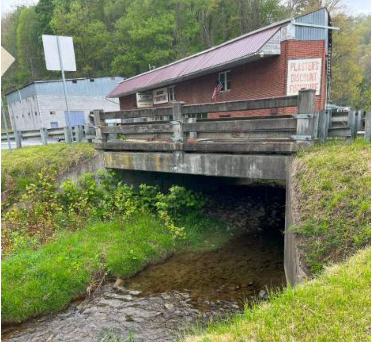
Figure 727: Culvert crossing Mill Creek
