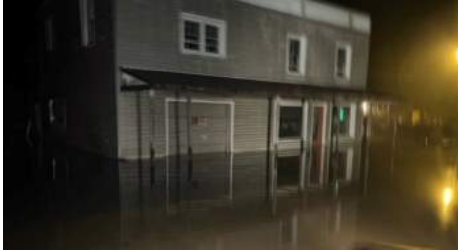
Figure 624: Flooding in Bandy, VA in July 2022 40
