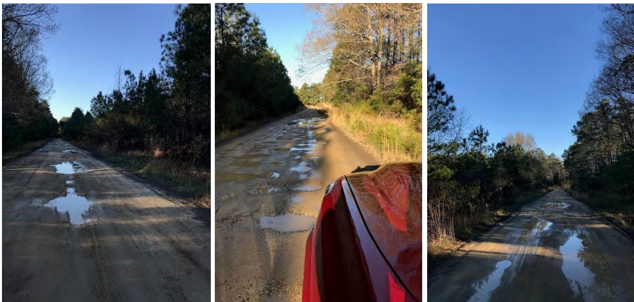
FIGURE 10: PHOTOS OF PUBLIC ACCESS ROAD LEADING TO CAPTAIN SINCLAIR'S.
