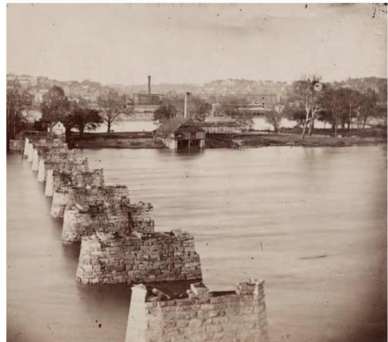
Ruins of Mayo's Bridge (1865)
