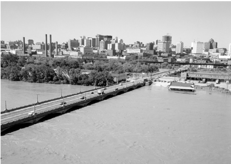
Mayo Island – floodwaters of Hurricane Camille (1969)
