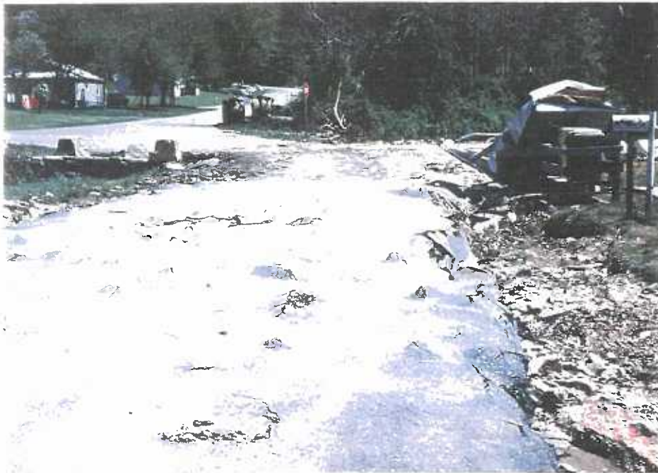
Destruction of 12th Street from Noels Run in April 1992.
