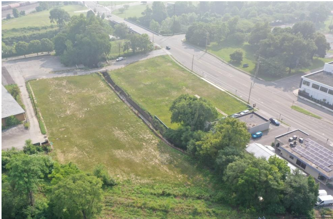
(B) Post Demolition – June 29, 2023
