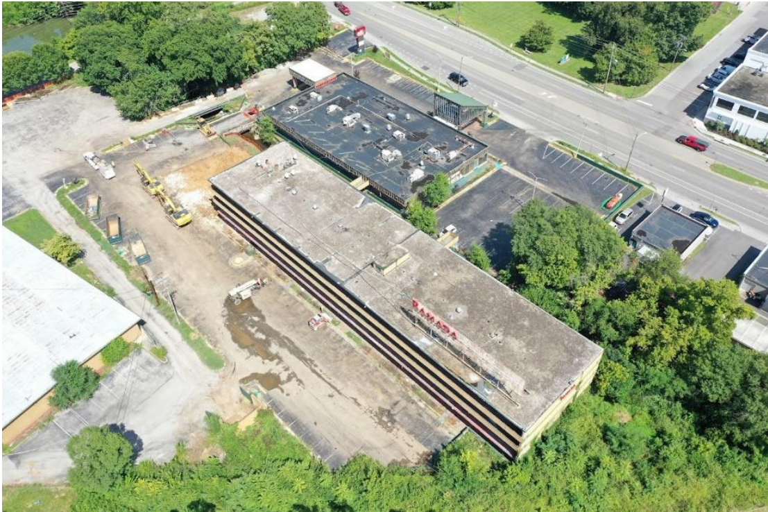
(A) Pre Demolition – Aug 17, 2022
