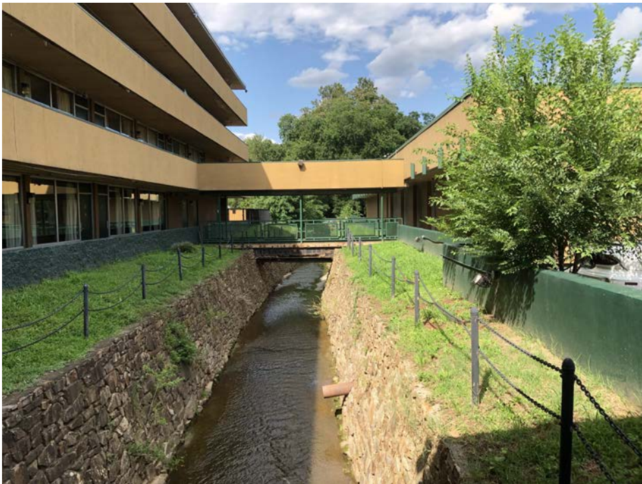
Facing Upstream on Ore Branch (Pre-demolition Photo)
