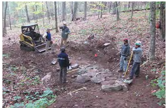
Work crews installing a drainage feature. Courtesy of IMBA/Rich Edwards.
