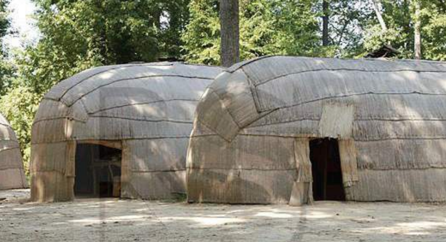
Reconstruction of a longhouse, showing ovoid form produced by the bent saplings and woven mat cladding
