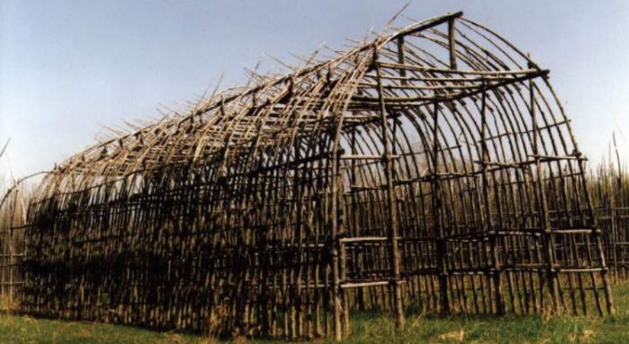
Reconstruction of a longhouse, showing sapling framing
