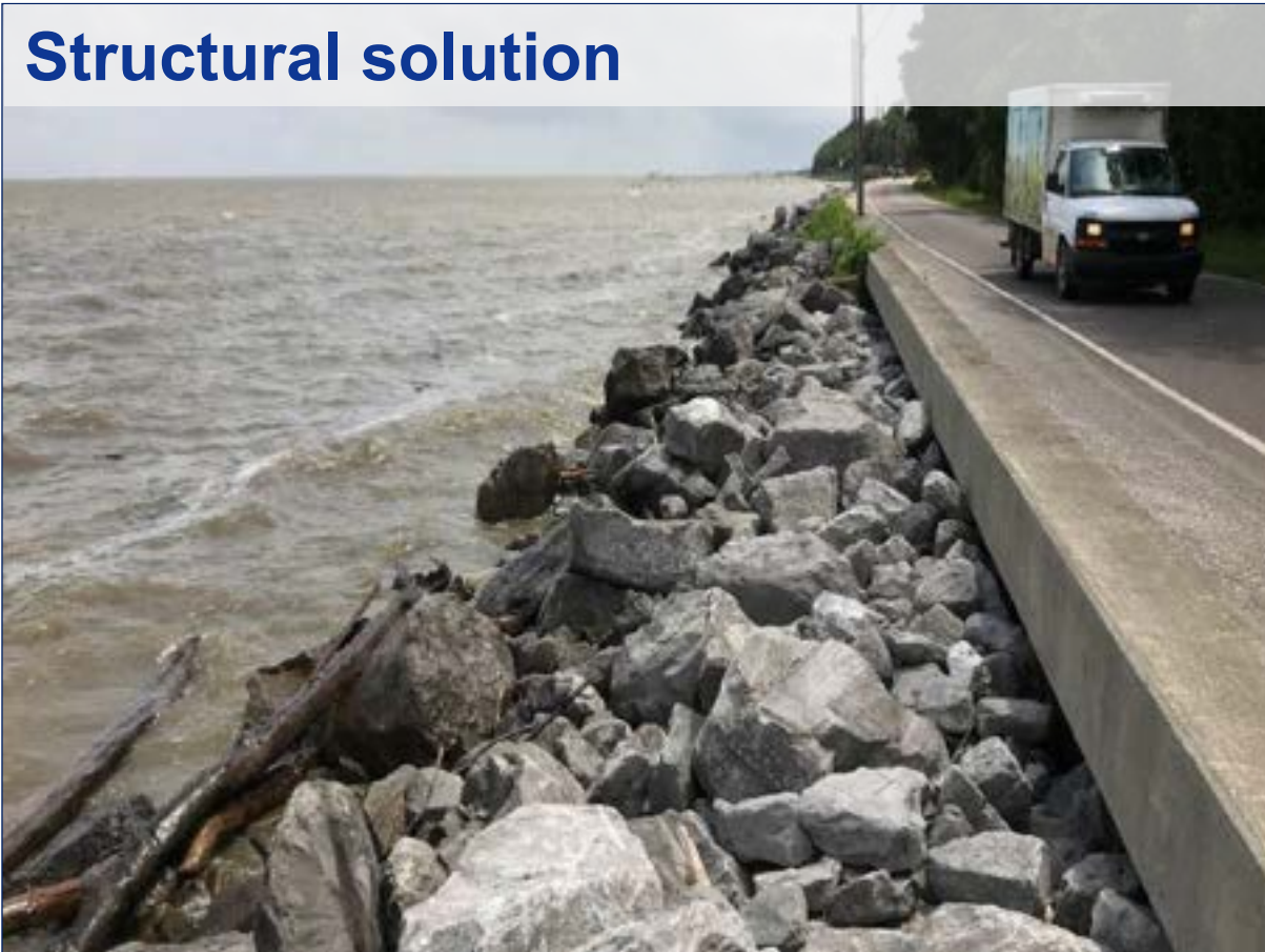
Traditional Seawalls: concrete and riprap
