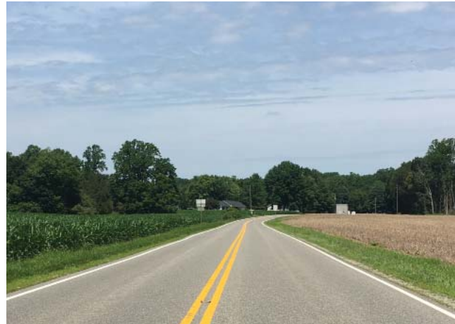
Minor Arterial, Dutton Road (Route 198) Source: Gloucester Planning and Zoning
