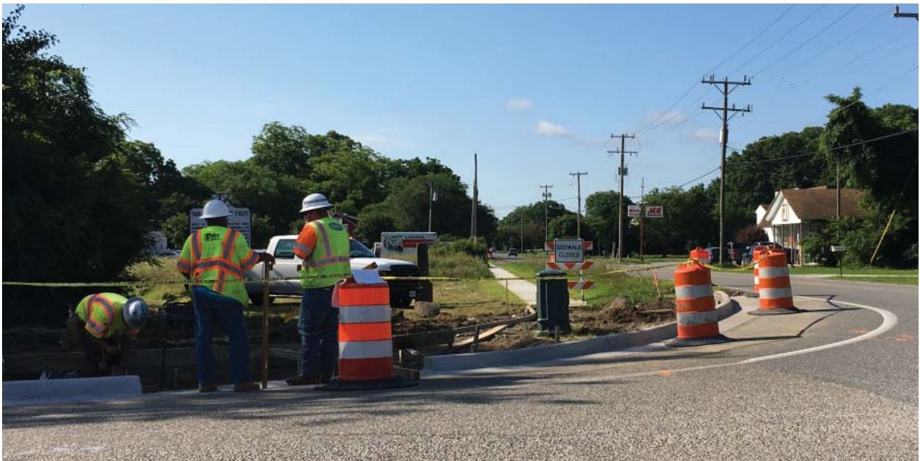
Construction of the Hayes Road Sidewalk - Source: Gloucester Planning and Zoning
