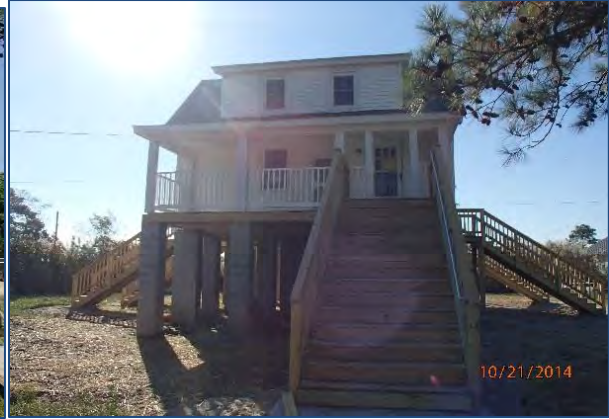
Figure 76: House in Hayes, Gloucester County - AFTER elevation.
