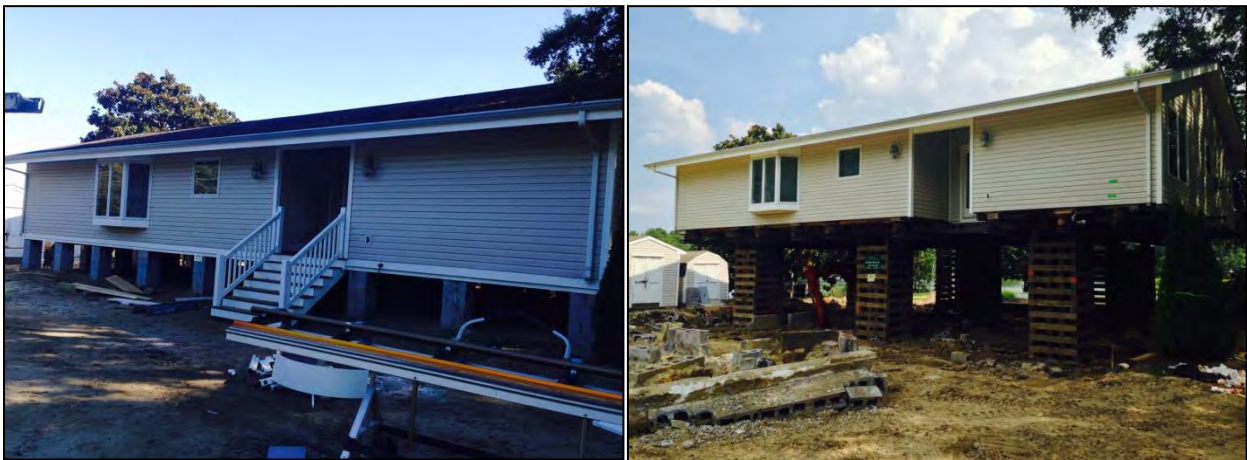
Figure 82: Photos of an elevated home in Port Haywood during (left) and after (right) being elevated (Mathews County, 2015).
