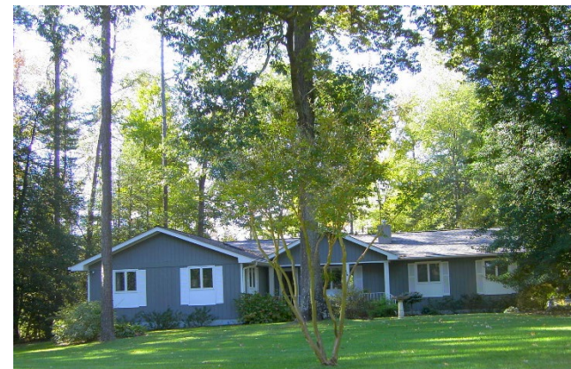
Queens Creek Residential
