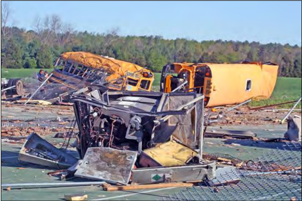
Figure 14: Photo of the damage at Page Middle School in Gloucester County (Gloucester-Mathews Gazette Journal, 2011).
