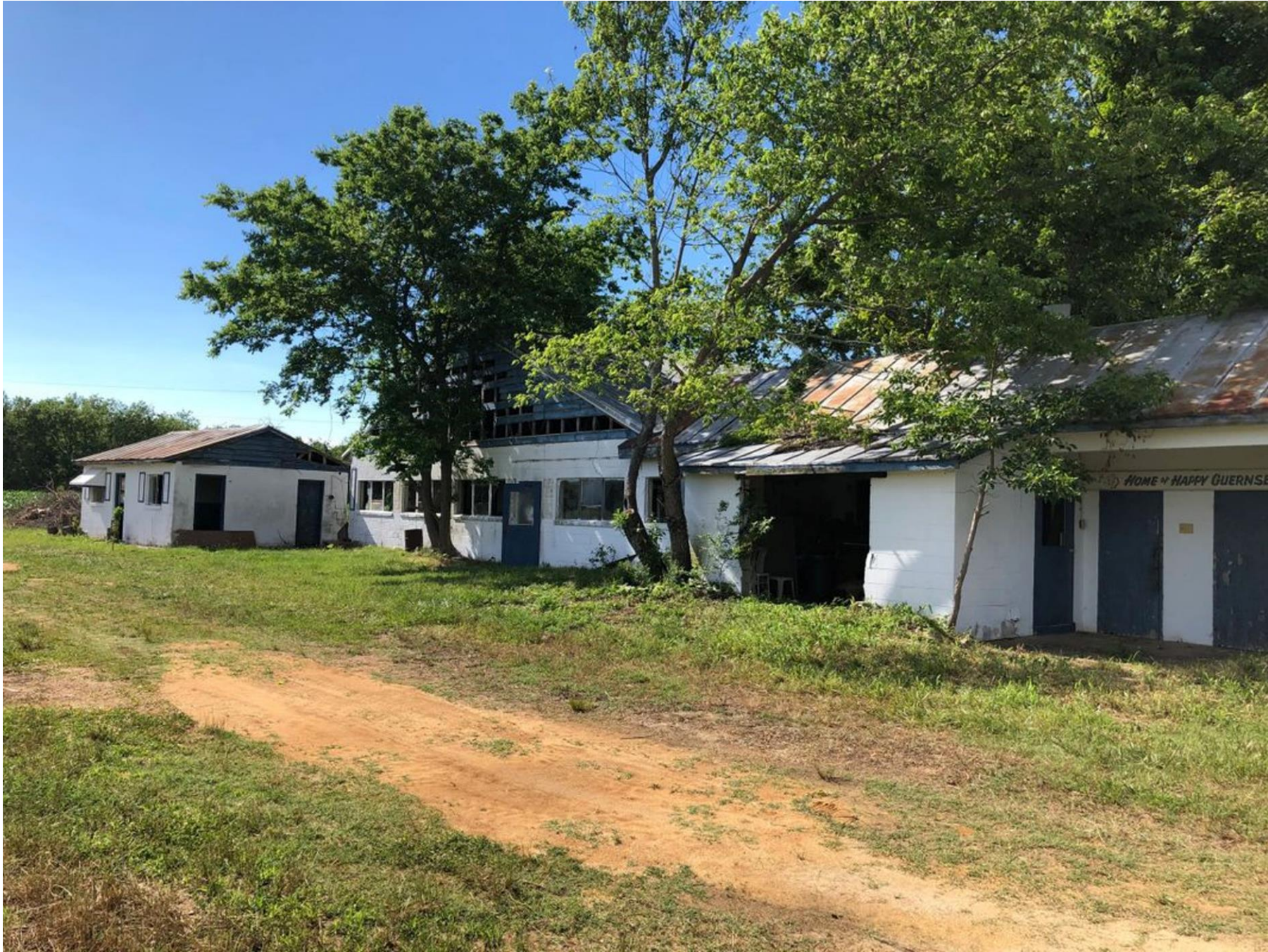
Farm buildings on Bushy Park Farm used when the property was a dairy farm.
