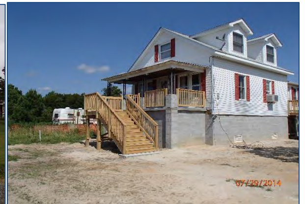
Figure 80: House in Hayes, Gloucester County - AFTER elevation.
